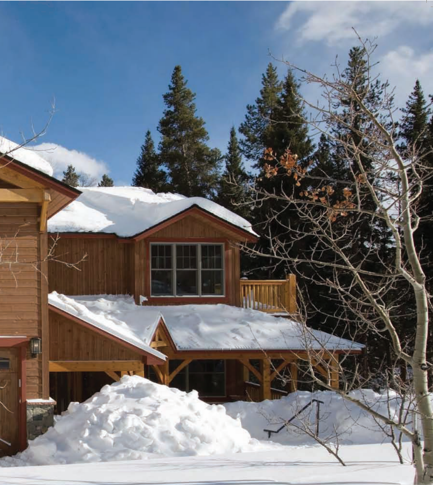
Mounds of snow shoveled from the roof all but obscure the front entrance of the Speares' home in Colorado's ski country. For efficient insulation, Woodhouse wrapped the home in structural insulated panels (SIPs) manufactured by Murus. A corrugated metal roof mimics the style used on old Colorado mine buildings.
