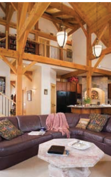
ABOVE: Gracefully curved knee braces support the trusses. Chad and Nancy opted for a timber frame cut from Douglas fir because its exceptional strength allows for longer spans to create a totally open great room.
