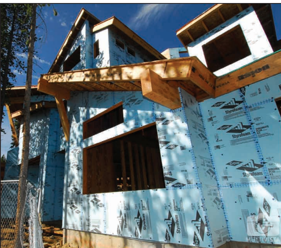
The exterior of this Breckenridge energy-conserving home is covered by one inch thick Styrofoam insulation to prevent heat loss, lower energy costs, and reduce associated CO 2 emissions.
